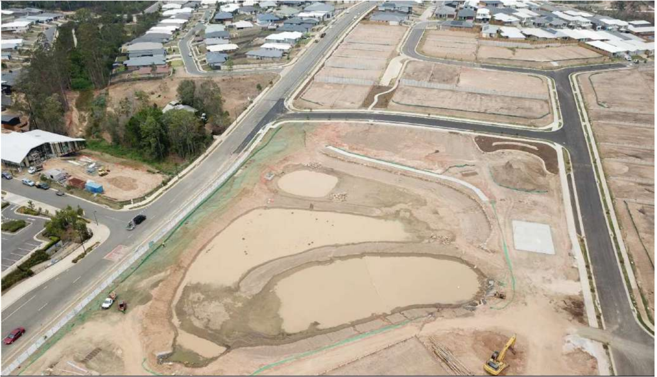
Photo 4: Aerial view of Stage 2 Wetland Construction– December 2019
