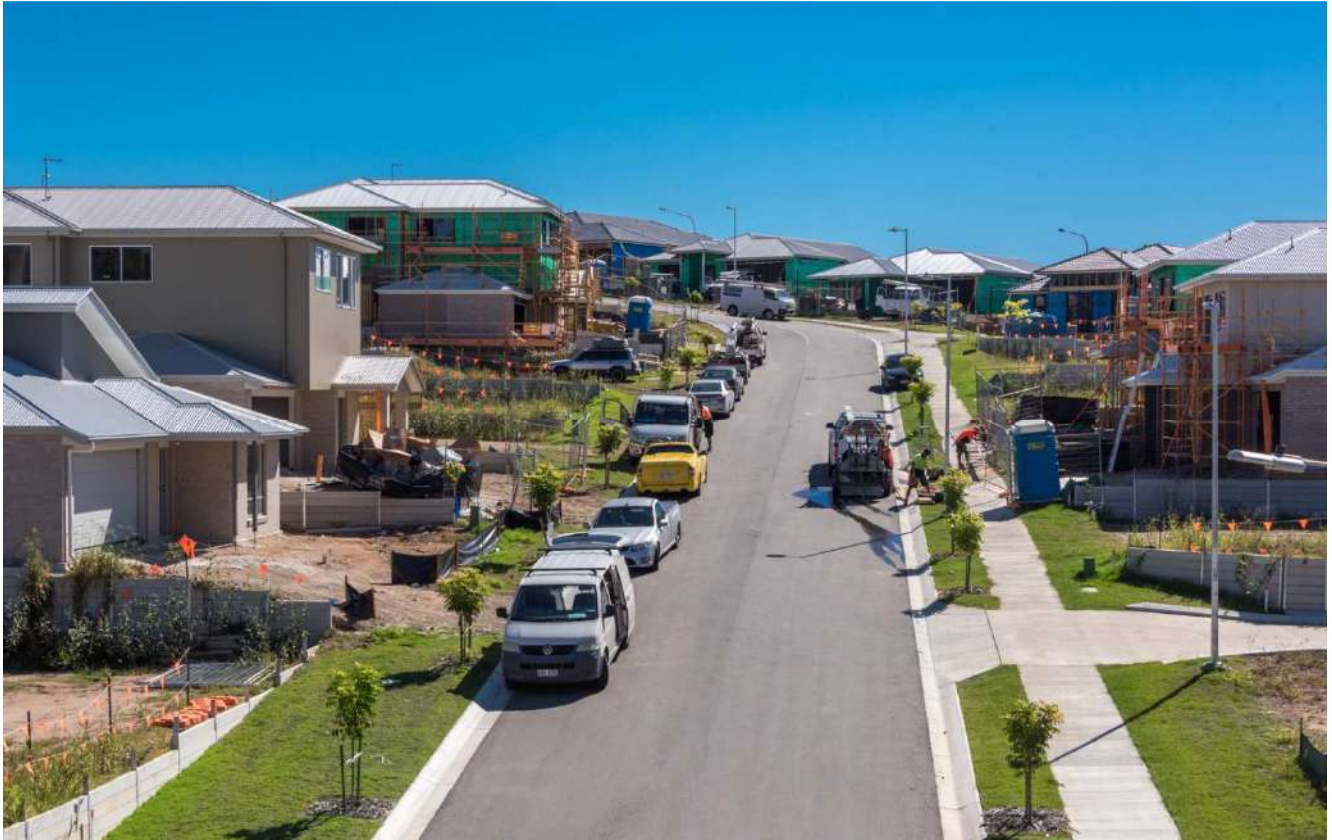
Photo 8: Stage 1 Housing – December 2019
