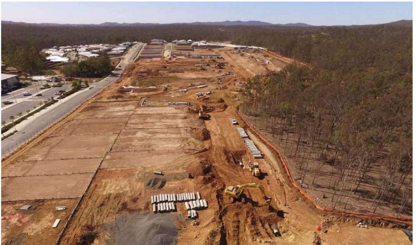
Photo 3: Aerial view of Stage 2 – Civil construction August 2019
