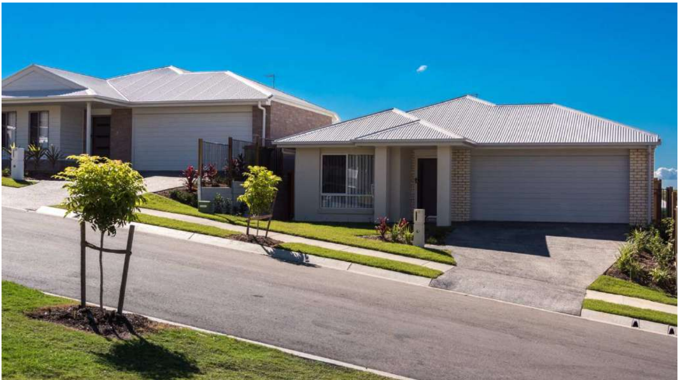
Photo 7: Stage 1 Housing – December 2019
