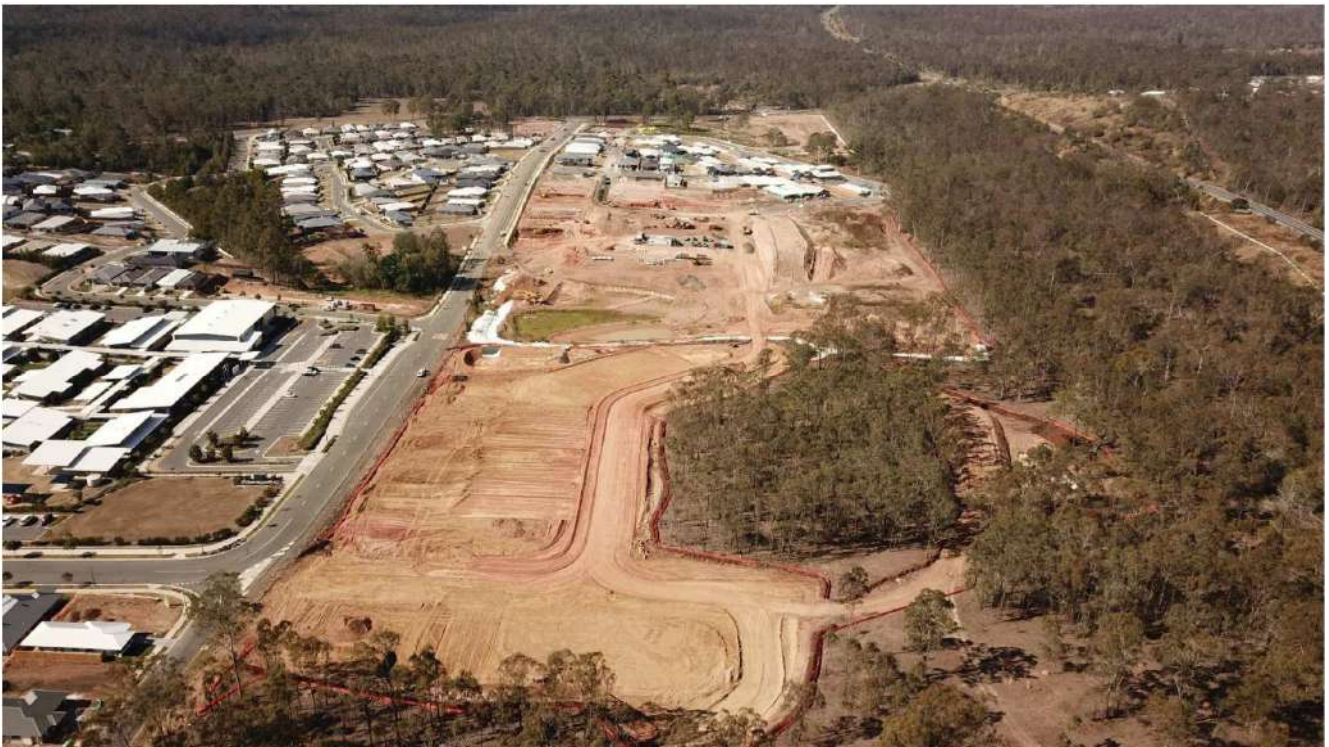
Photo 1: Aerial view of Stage 2A-Stage2D - June 2019
